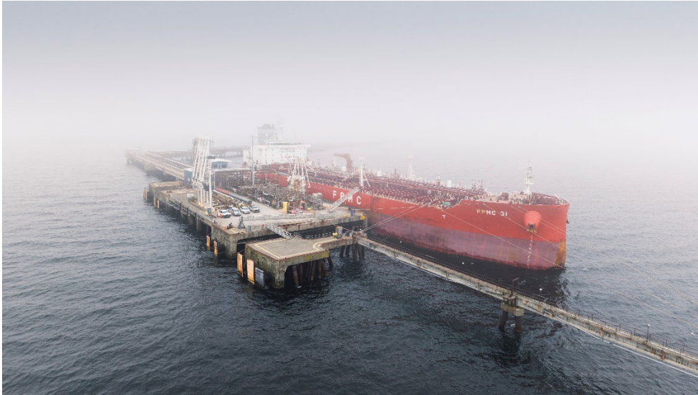
Vessel docked at Braya's jetty
